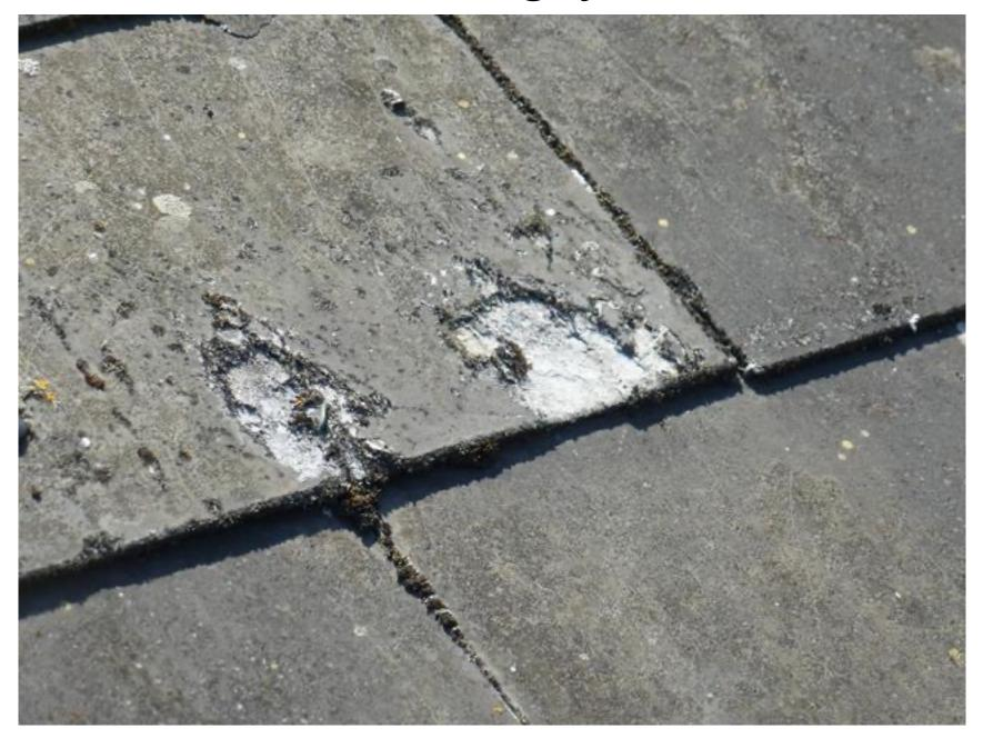
Slates are friable and can be easily broken.
